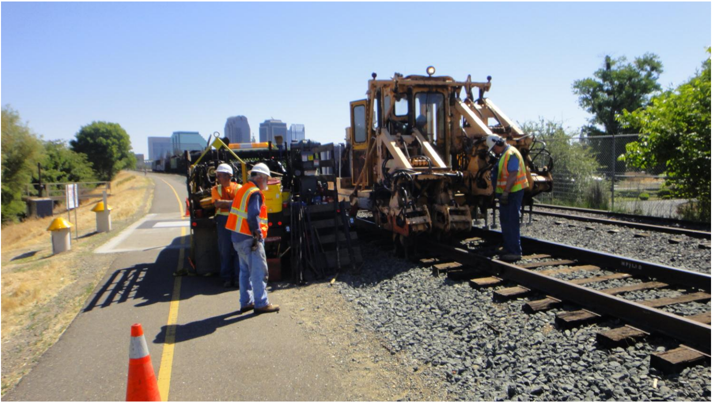
Tamping the newly installed rail.
